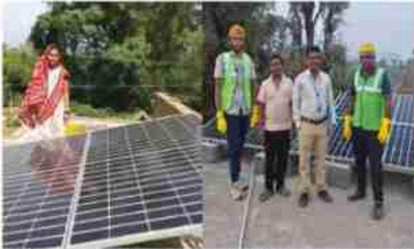
A woman beneficiary of PM Surya Ghar Muft Bijli Yojana (left). On the right, engineers install a rooftop solar power unit in Odisha's Ganjam district. — Image by Aishwarya
